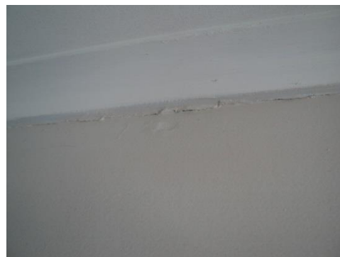
Photo 18– Typical 'tearing' of joints due to slab and framing movement.
