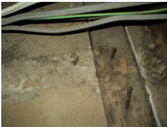
Photo 15- Fully destroyed ceiling battens
