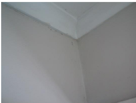
Photo 17 – Typical 'tearing' of joints due to slab and framing movement.
