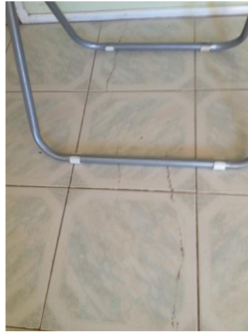
Photo 14 – Multiple split tiles due to slab cracking
