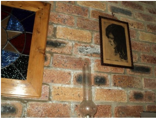
Photo 9- Moisture effervescence to bricks.
