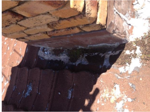
Photo 8- Re-patching to chimney flashing
