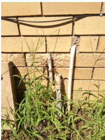
Photo 11- Spot fretting of brickwork
