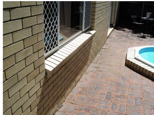
Photo 4 – Moss/staining to base of wall.
