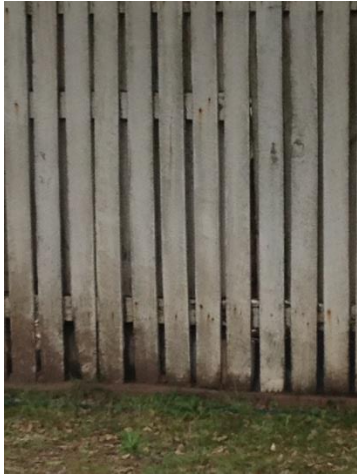
Photo 1 – Rot to batten bases and posts
