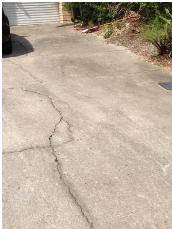
Photo 3 – Moderate movement cacking
