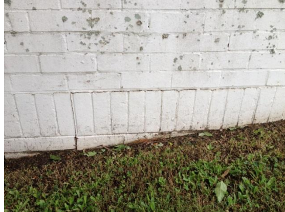
Photo 2 – Returned cracking to brick base
